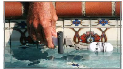
3. Once the valve with the 3" gray plastic tube are glued into the fill line, fill the pool or spa up to the desired level with a garden hose and then turn the hose off. Turn the fill line water valve on just/turn, you don't need much pressure for the valve to do its job. Adjust the float to the desired level. Remove the two stainless steel screws on the 3" gray plastic tube at this time and set them aside.
